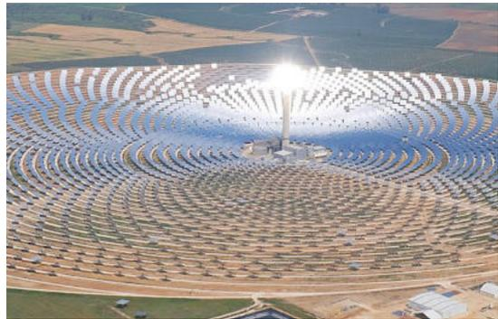
(a) Solar panel (b) Solar power tower or solar concentrator situated in Spain. Here the heat energy of the sun is condensed and utilized by using curved mirrors.
